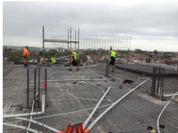
(b) Typical floor – manual placement of SL102 mesh sheets
