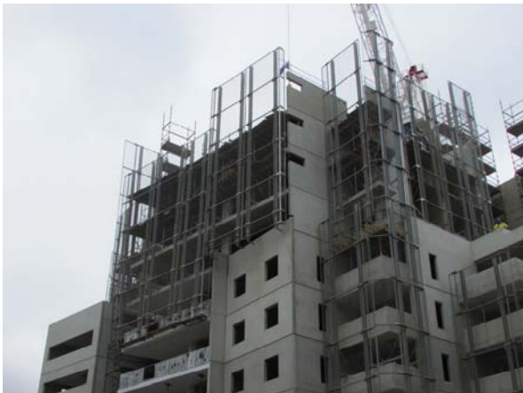
(a) External precast concrete panel façade
