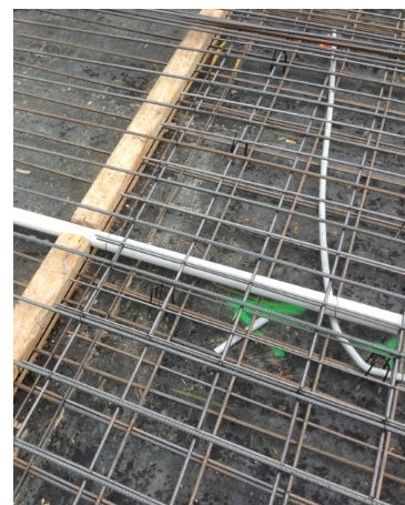
(e) Typical floor – mixed steel at pour joint
