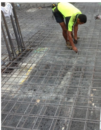
(c) Typical floor – chairing mesh sheets
