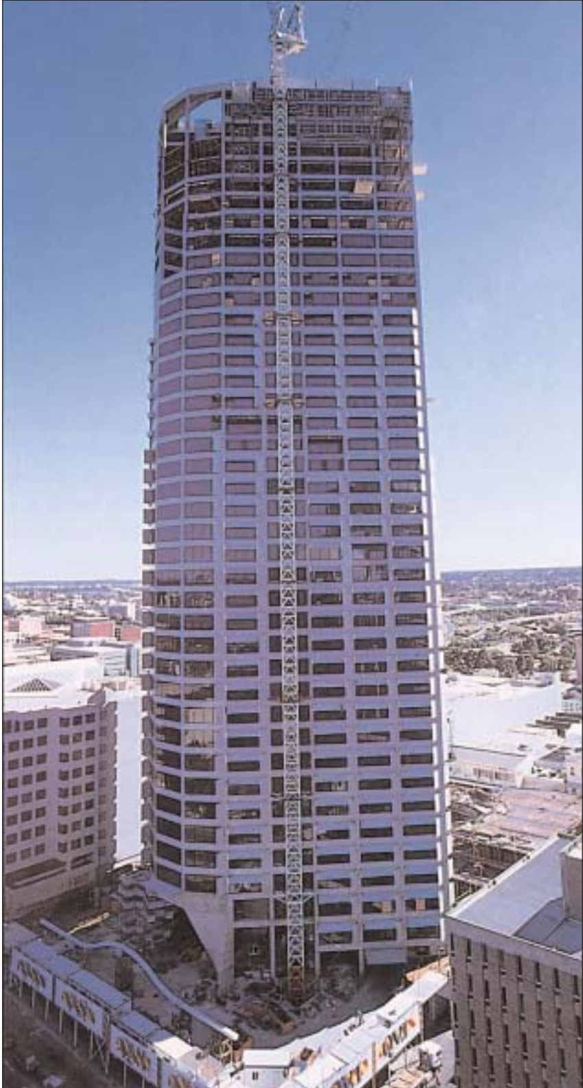
Construction progress: mid-April 1999
