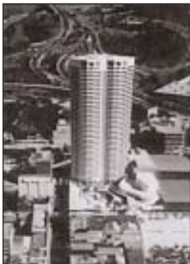
The slipform ran at speeds of up to 600 mm per hour
