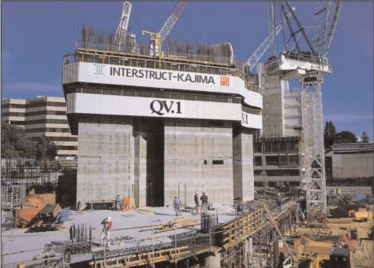
The slipform ran at speeds of up to 600 mm per hour
