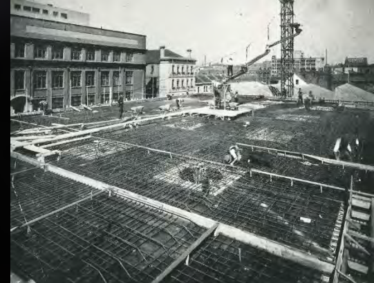
Flat slab floor to garage (A.R.C. Reinforcements)
