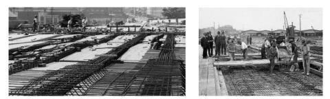
Figure 5. Monier System with bars bent into the top or bottom of the slab/beam (left) and concrete placement (right) on Eddy Avenue Bridge, Sydney, 1925 (ARHS RRC517458 left and 517470 right)
