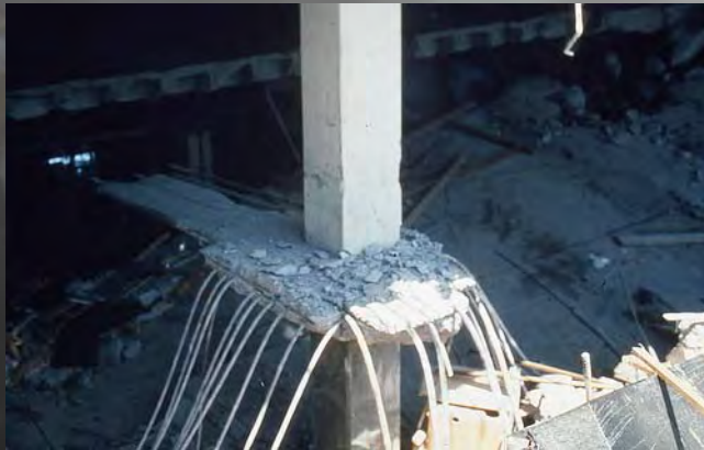
Remains of car park floor – Old Newcastle Workers Club NSW - Brittle failure & progressive collapse (Photo courtesy Cultural Collections, The University of Newcastle, Australia)
