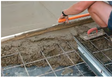
Figure 10 Formed control joint using pressed metal key joint profile
