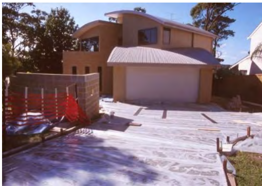
Figure 8 Clear plastic recommended for curing
