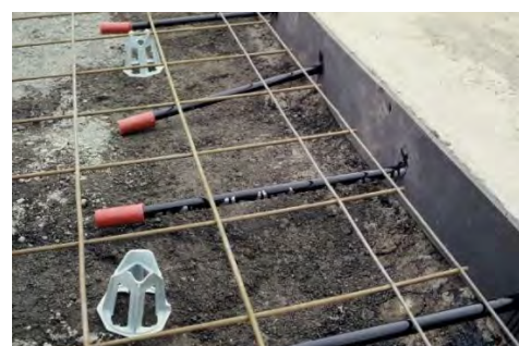
Figure 16 Ensure dowels are properly coated and aligned
