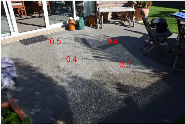
Figure 3 Example of cracking to patio slab
