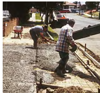
Figure 3 Reinforcement must be chaired at the correct height prior to placing concrete
