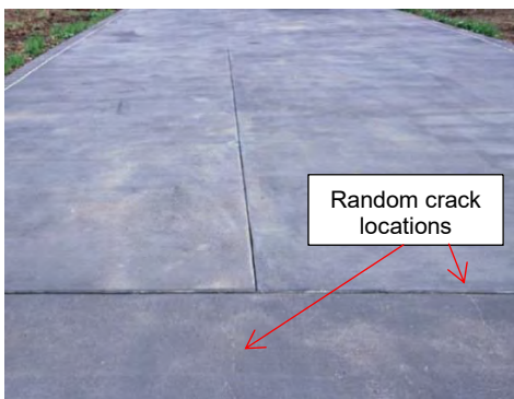
Figure 12 Ensure joints are continuous
