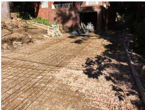
Figure 3 Reinforcement must be chaired at the correct height prior to placing concrete
