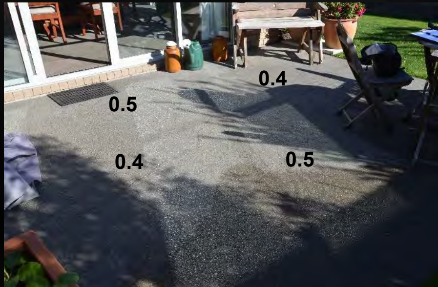
Cracking unacceptable to owner
