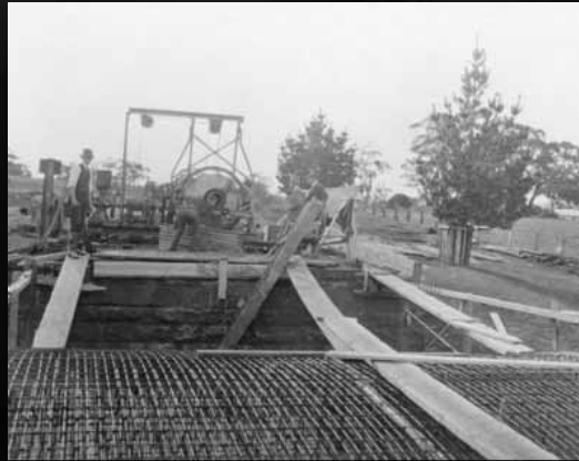
Construction of Wannon Bridge, Ararat, Victoria, 1917
