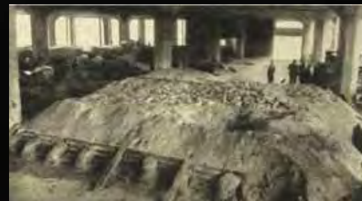
13.5 Tons (23.5kPa) Test loading of the Innes-Bell flooring system on the Smith and Waddington's Limited Factory, Camperdown, NSW, circa 1927. Deflection of 1/16 in. (1.6 mm)
