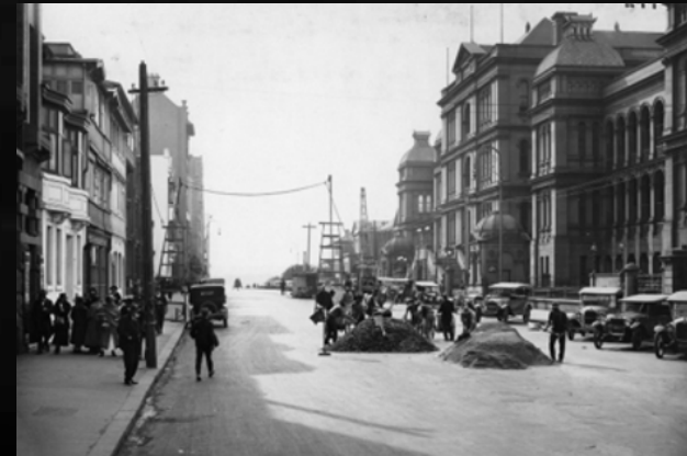
Hand-mixing concrete in Clarence Street, Sydney, 1924
