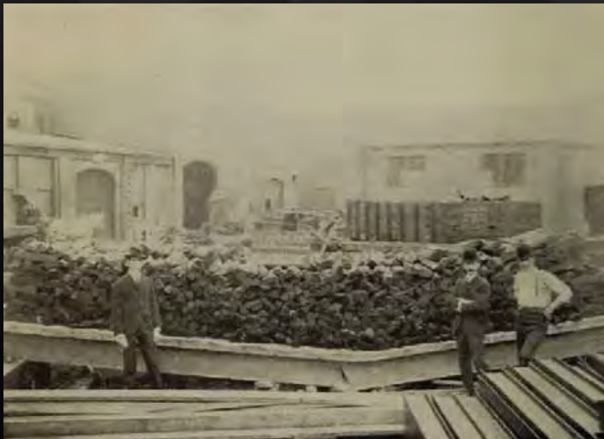
Failure of two Kahn reinforced beams
