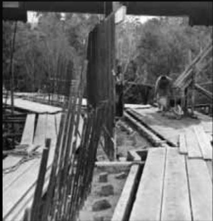
Square bars and key stones Nambucca Heads, NSW 1950s
