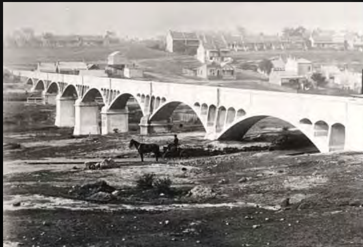
Johnstons Creek Sewer Aqueduct Annandale, Sydney (1896)
