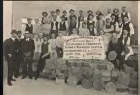
35 Tons Load testing of completed reinforced concrete floor of the Sniders and Abrahams warehouse, Melbourne, 1909 Deflection 3/16 in.
