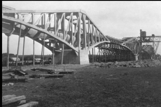
Geelong Sewage Aqueduct, 1914
