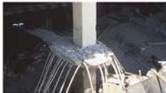
**Figure 1** Punching shear failure with structural integrity reinforcement preventing collapse of slab, Hotel Grand Chancellor, Christchurch
