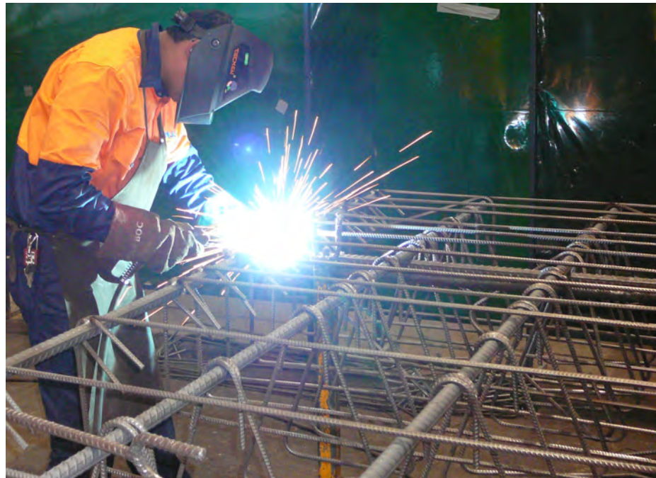
FIGURE 8 Welding provides for safe, accurate assembly of column and beam reinforcement
