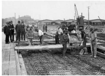
**Figure 5. Monier System with bars bent into the top or bottom of the slab/beam (left) and concrete placement (right) on Eddy Avenue Bridge, Sydney, 1925 (ARHS RRC517458 left and 517470 right)**
