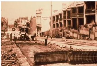
**Figure 6. Rolled mesh used on Walker Street, North Sydney**
