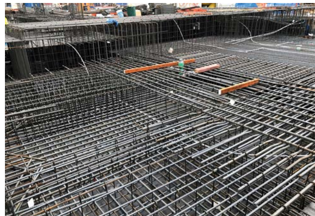
Figure 3 Typical surface condition of reinforcement on site
