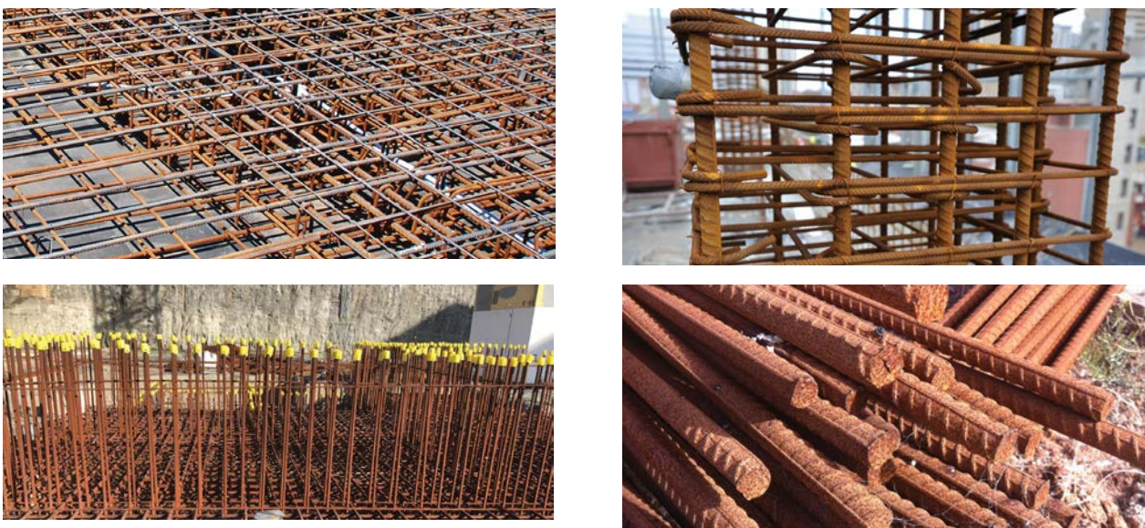
Figure 1 Examples of acceptable surface condition of reinforcement
