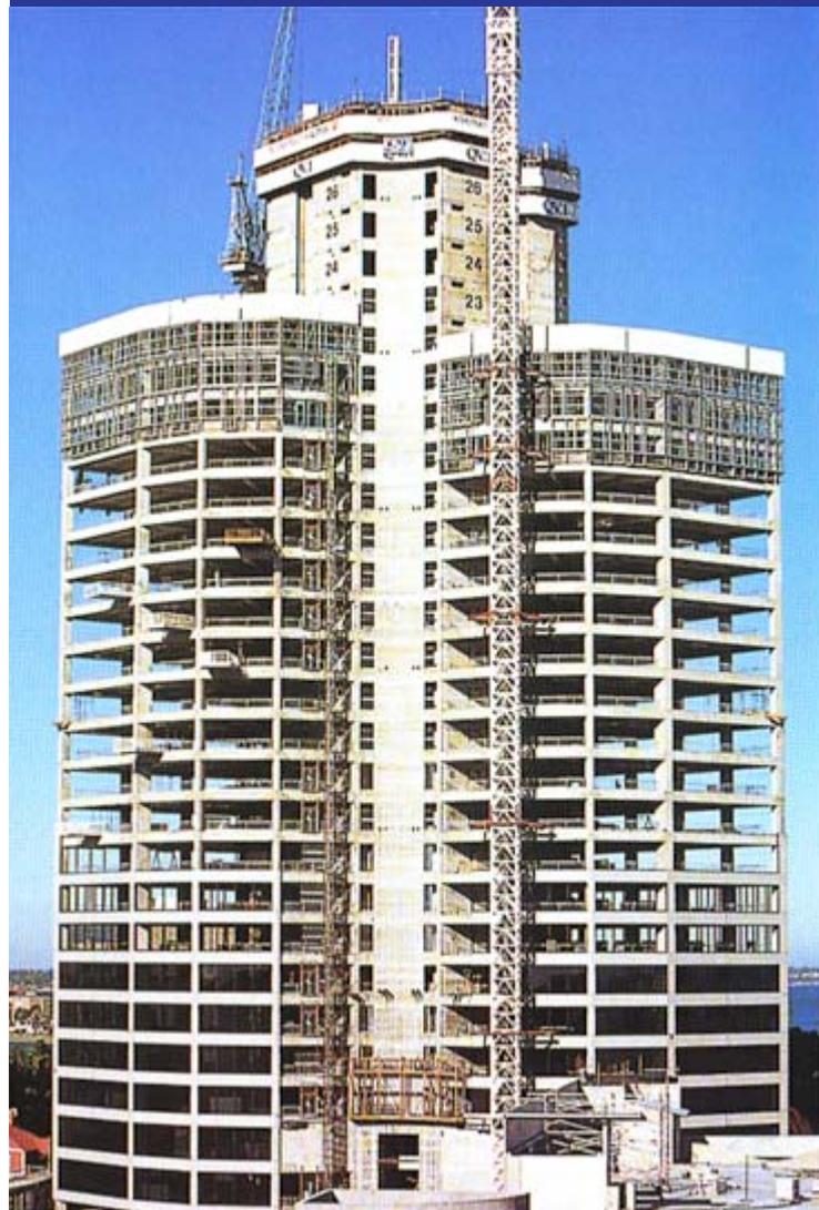
*Typical Concrete Building Frame – economical, fast to construct and minimum storey heights.*
