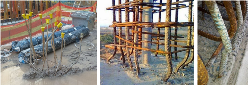
Figure 10 Examples of bending reinforcement on site
