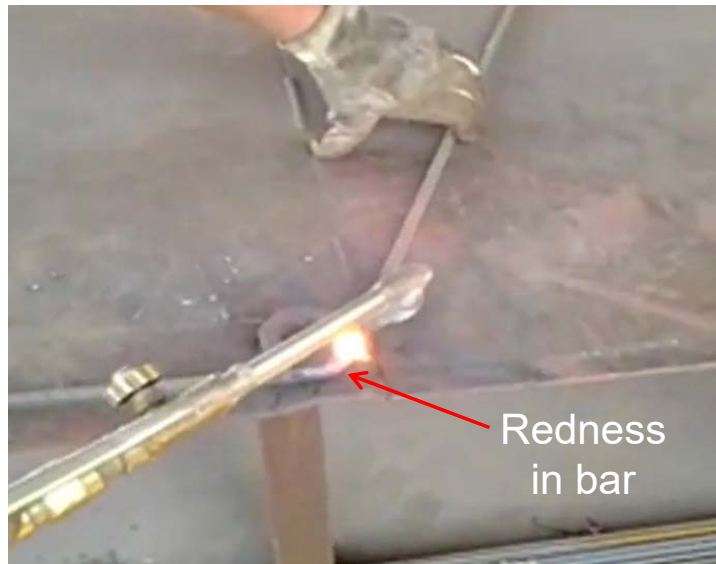
Bar overheated based on steel colour
