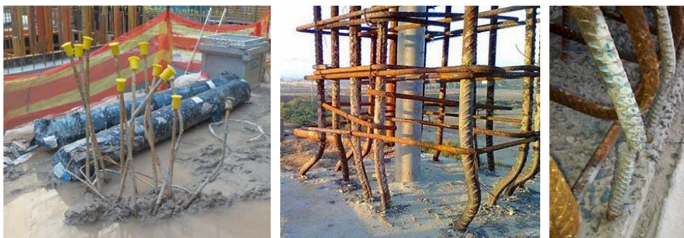
Figure 10. Examples of bending reinforcement on site.
