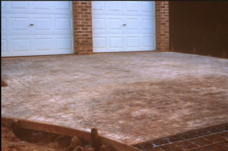
Efflorescence
