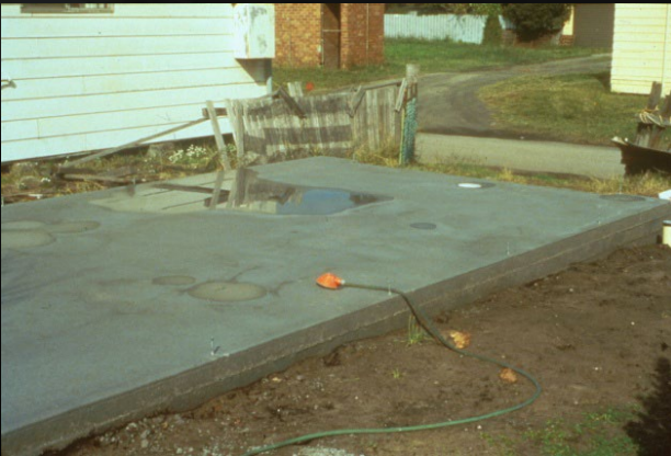
Add water to concrete (must be continuous)
