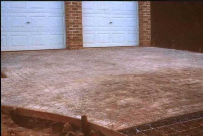
Efflorescence
