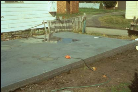
Add water to concrete (must be continuous)
