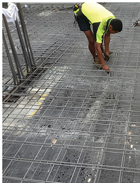
Figure 1 Suspended concrete floor construction using Ductility Class L mesh
