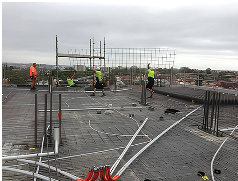
Figure 1 Suspended concrete floor construction using Ductility Class L mesh
